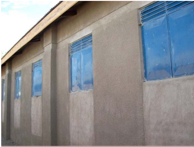
Exterior Dormitory Walls
